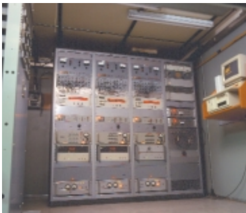
Figure 3.6. WWV Control Room
