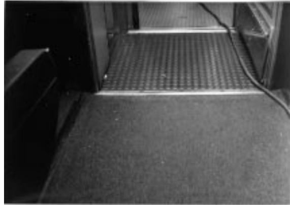
**Figure 3-2. Carpet and Resilient Rubber Floor Covering**
