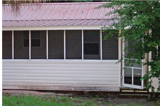
Figure 5-3: Floodwaters reached just under the first floor on this building (photo courtesy of AECOM)
