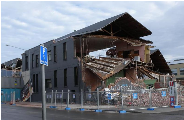
Figure 5-1: Failure of unreinforced masonry wall during an earthquake event. (Photo courtesy of Degenkolb Engineers)
