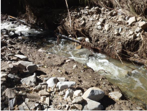
Figure 9-10. Exposed and Broken Distribution Lines Resulting from Flooding in Jamestown, CO (Courtesy of David Goldbloom-Helzner)
