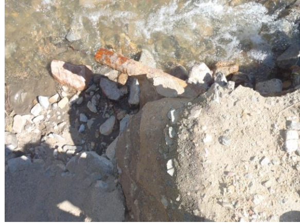
Figure 9-10. Exposed and Broken Distribution Lines Resulting from Flooding in Jamestown, CO (Courtesy of David Goldbloom-Helzner)
