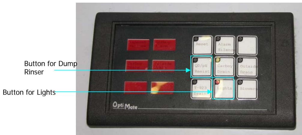
2. Select the desired dump rinser program and adjust the program parameters. All of the programs use a dump period, which is the amount of time that the dump door is open. However, the techniques used to determine when the tank is full and when a run is completed varies.
