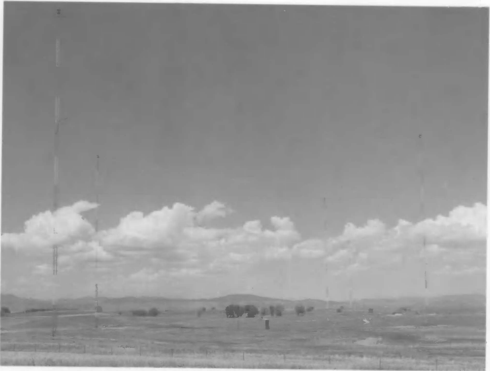
Facilities near Fort Collins, Colorado, for stations WWVL and WWVB. The antenna for each station consisted of four steel towers arranged in a diamond 1900 feet long and 750 feet wide.
