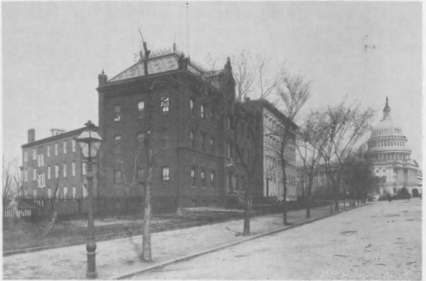
The Coast and Geodetic Survey building, home of the Office of Weights and Measures, in the 200 block of New Jersey Avenue, S.E., as Dr. Stratton saw it in 1900. The Butler building, into which the new Bureau of Standards expanded, is probably the structure next door. "Bushey House," at 235 New Jersey Avenue, is out of the picture, down the street.
