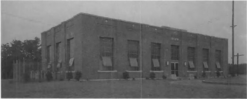
Exterior of NBS radio broadcasting station WWV, Greenbelt, Maryland. From this station, standard radio frequencies of 2.5, 5, 10, 15, 20, and 25 Mc were transmitted continuously. Two standard audio frequencies, 600 and 400 cycles, were broadcast as modulations on each radio frequency.
