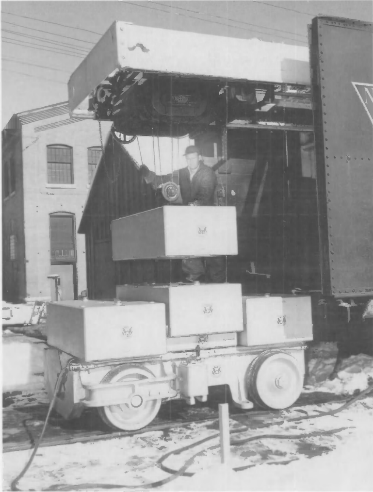
Although NBS had no regulatory duties or power to initiate investigations, if called upon it could serve as an impartial arbiter. Here, Charles H. Oakley lowers a 10 000 lb weight onto a railway-scale test-car in order to test the Union Pacific scale. In 1913, at the request of the Interstate Commerce Commission, NBS began testing railway scales. These scales were the source of continual complaints, and the railways, fearing for their reputations, were eager to rectify the situation.
