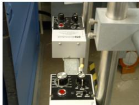
Chamber alignment controls 100 kV range
