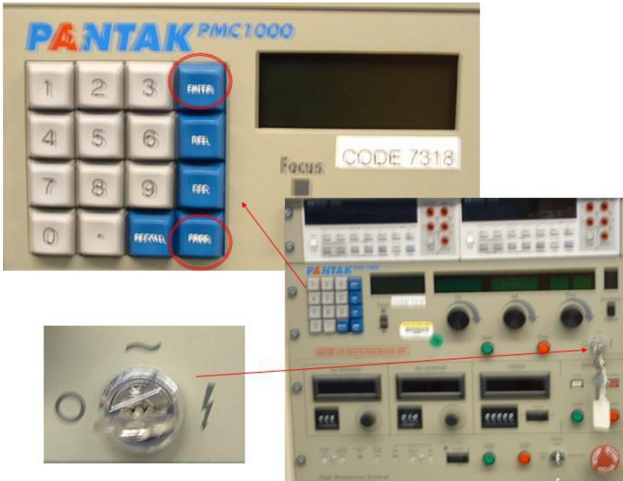
Figure 6. 100-300 kV x-ray controls.
