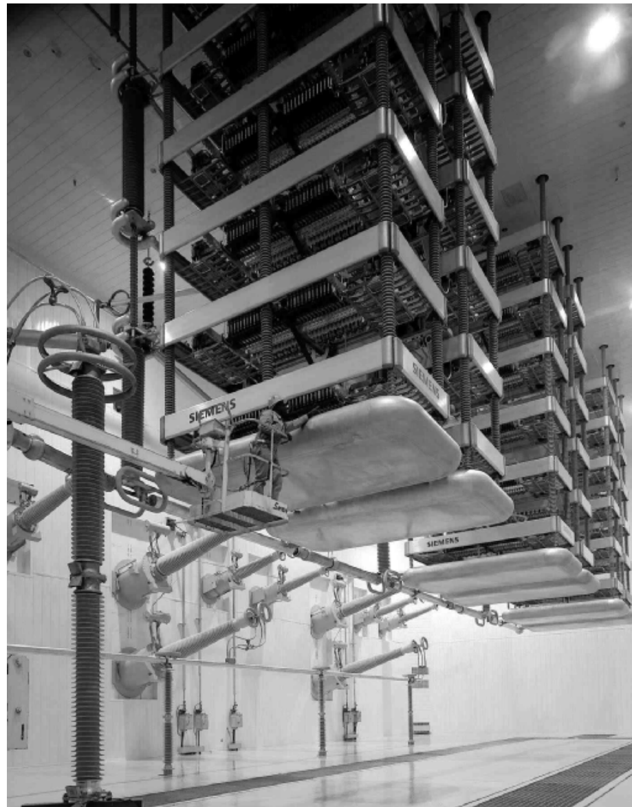
Suspended Thyristor Based Quadruple Valves making a 12-Pulse Converter rated 500kV (Pacific DC Intertie) (Siemens)
