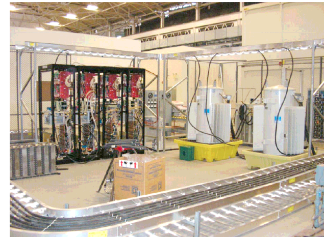
SSPS installed for testing at NSWC, Philadelphia (picture courtesy of NSWC & GE)
