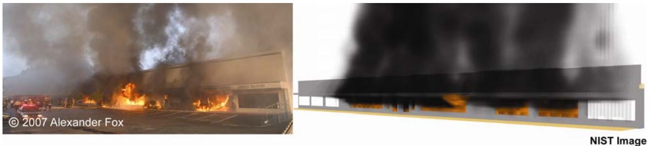
Figure 4-24. Comparison between photo and rendered image from the simulation at 1884 s (7:42:17 p.m.). The view is of the front of the main and west showrooms.
