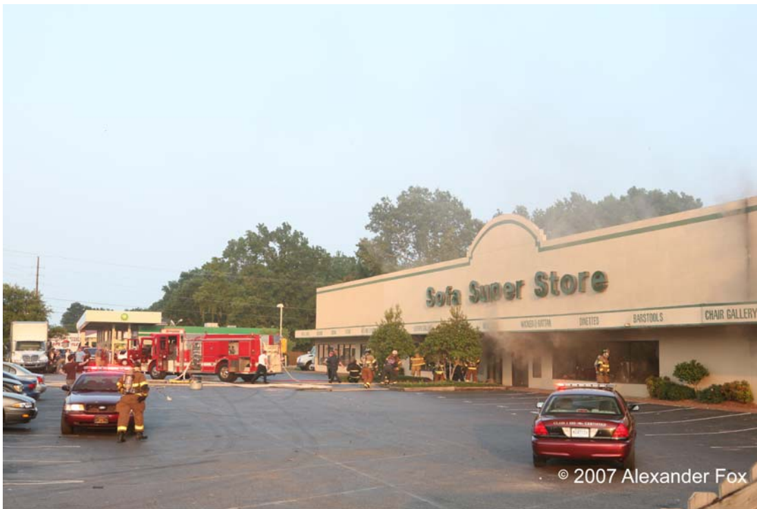
Figure 3-7. Light brown smoke began to flow out of broken front windows. Photo taken at approximately 7:35 p.m. Photo used with permission of Alexander Fox.
