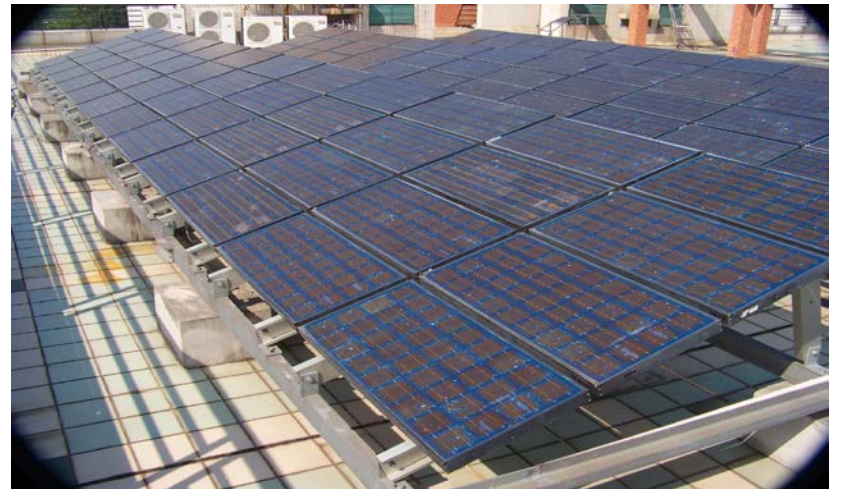
Re-installation of fielded Solarex modules
