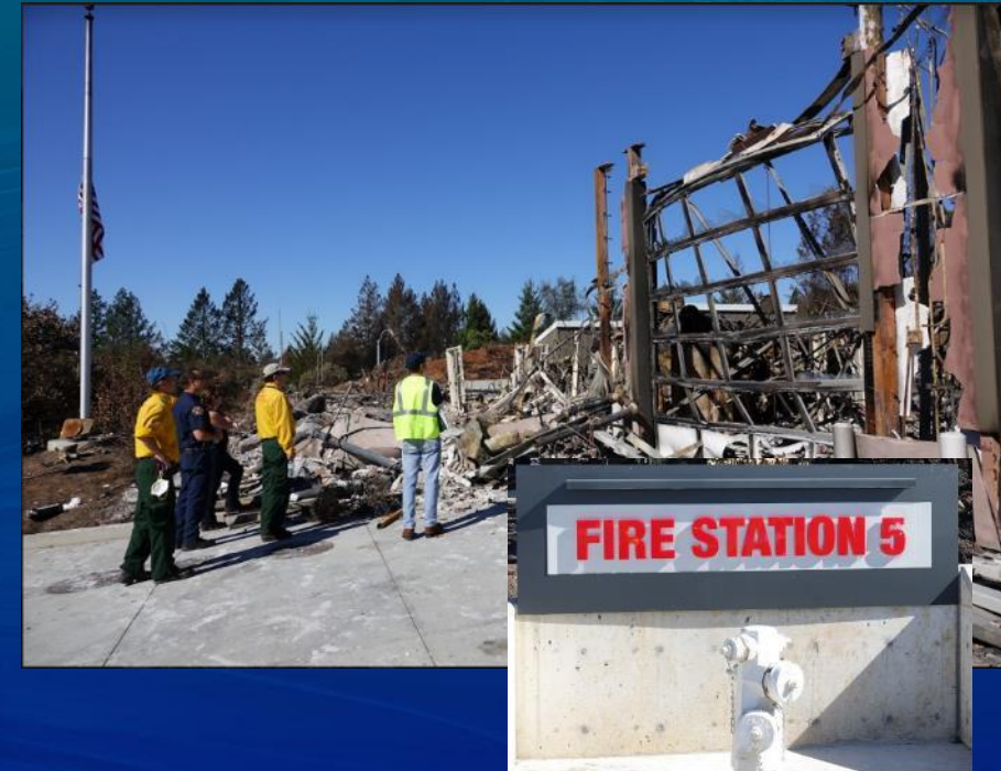
Destroyed Fire Station
