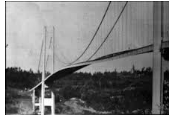
Tacoma Narrows Bridge (Galloping Gertie) opened in July 1940, but collapsed due to aero-elastic flutter four months later.
