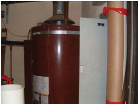
Natural Gas Hot Water Heater installed in Electrical Closet
