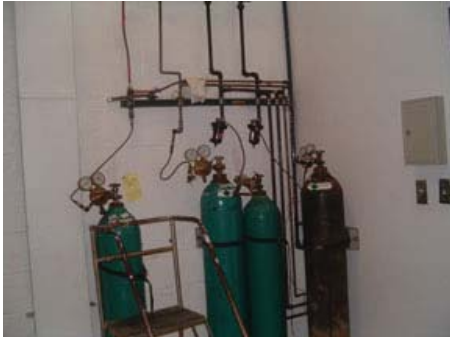
Laboratory Gases Manifold
