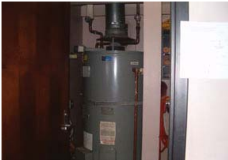
Natural Gas Hot Water Heater installed in Electrical Closet
