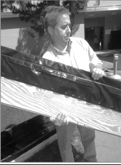
Exhibit 4. Showing how to hold a chute for the pour.
