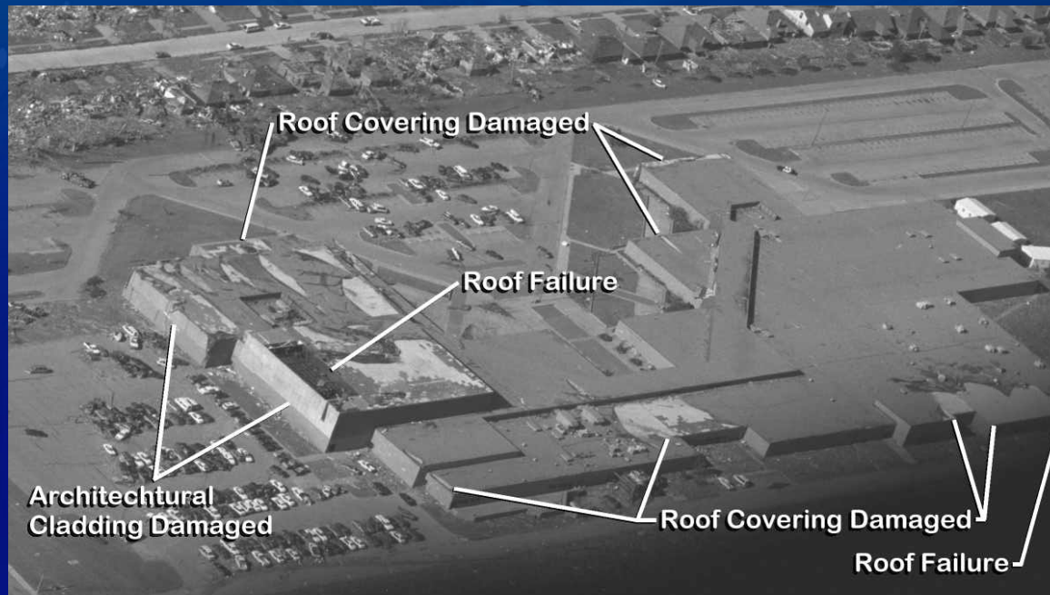
Aerial view of the damage done to Westmoore High School in Oklahoma, OK
