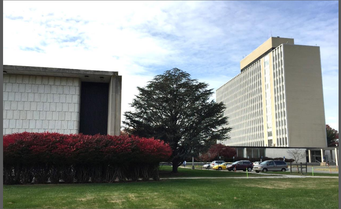
Building 101: Administration / Conference Center (1965)
