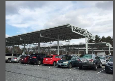
Parking / Solar Cover
