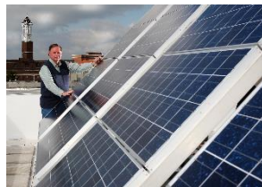
Solar Panels at Knoy Hall
