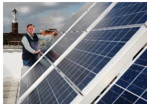
Solar Panels at Knoy Hall
