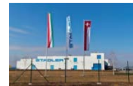
Stadler Szolnok 370 employees
