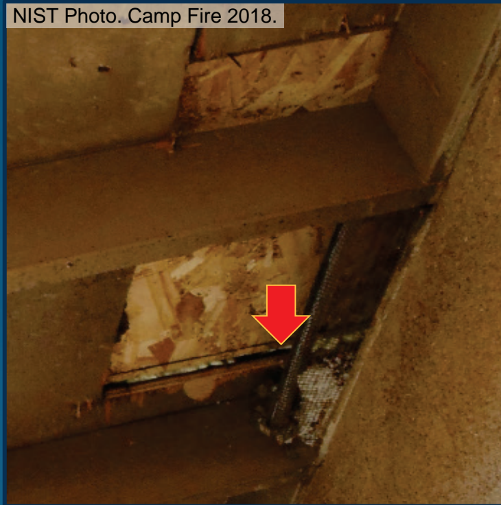
Failure: eaves/roof truss near eave vent
