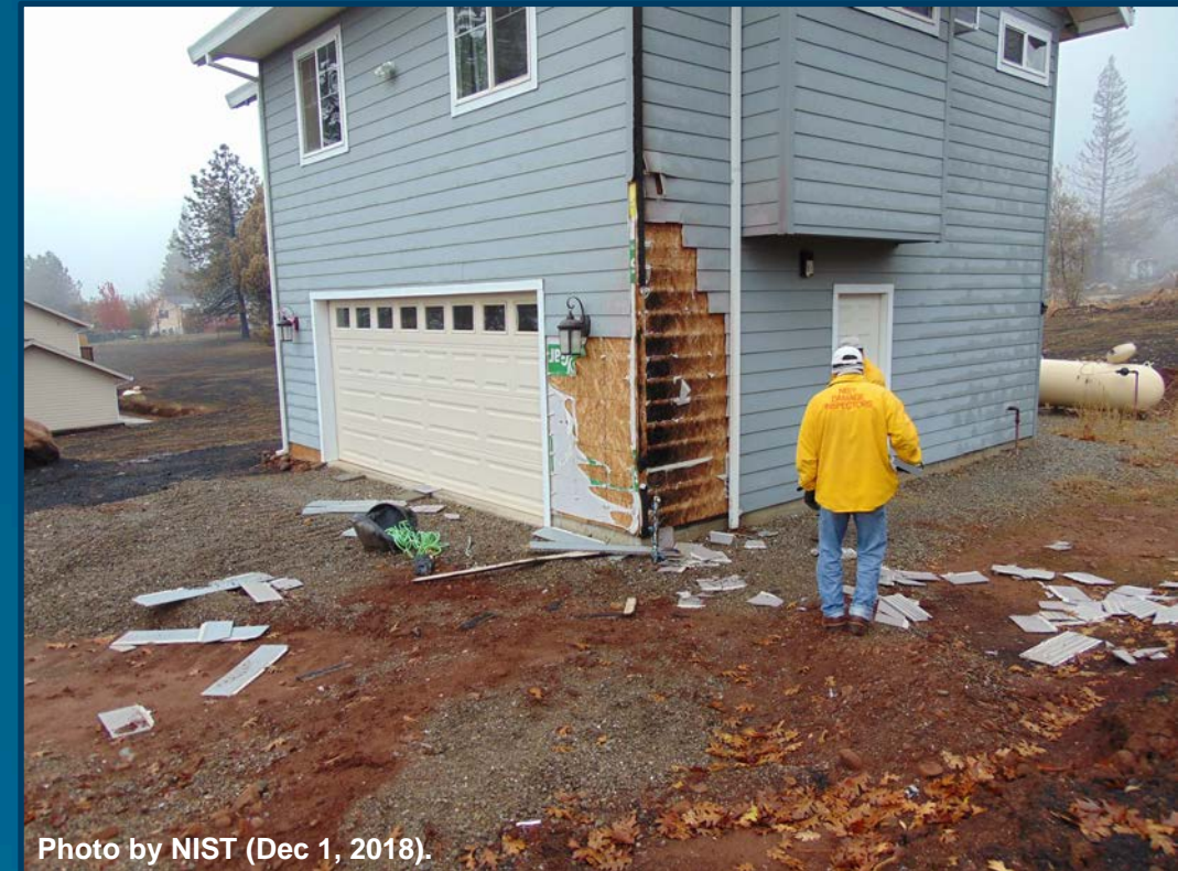
b) Associated evidence of the fire ignition and defensive actions encountered during NIST damage assessments.
