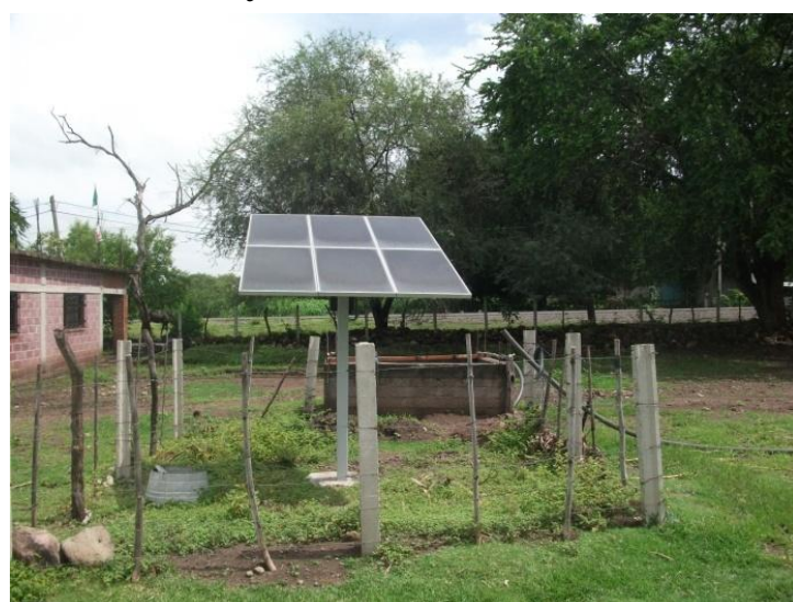
Figure 2. El "Amate" PV system array (2S x 3P). Array title angles: 22°
