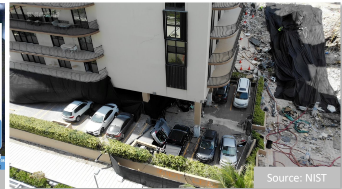
Eyewitness Accounts of Pool Deck Collapse
