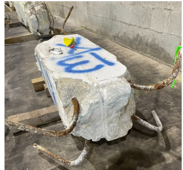
Same Column in Primary Evidence Facility
