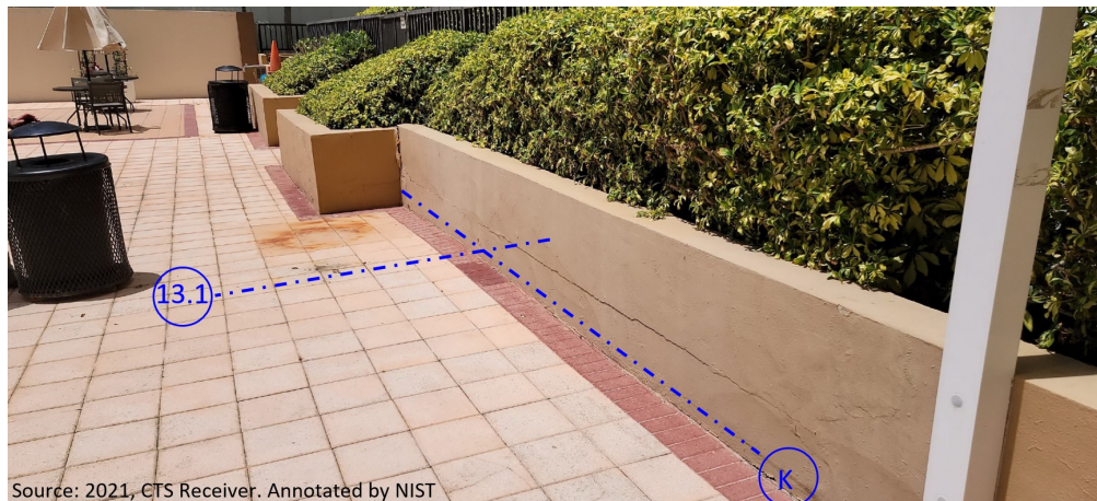
Damage to Pool Deck Planters Three Weeks Before the Collapse Indicated Severe Structural Distress
