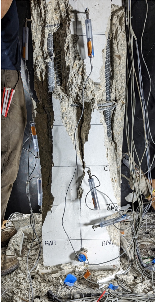
Left: specimen with short lap splice and sustained load
