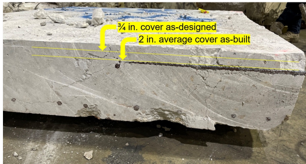
Top Reinforcement in Pool Deck Lower than Design Requirements Placement of Top Bars in Column Strips
