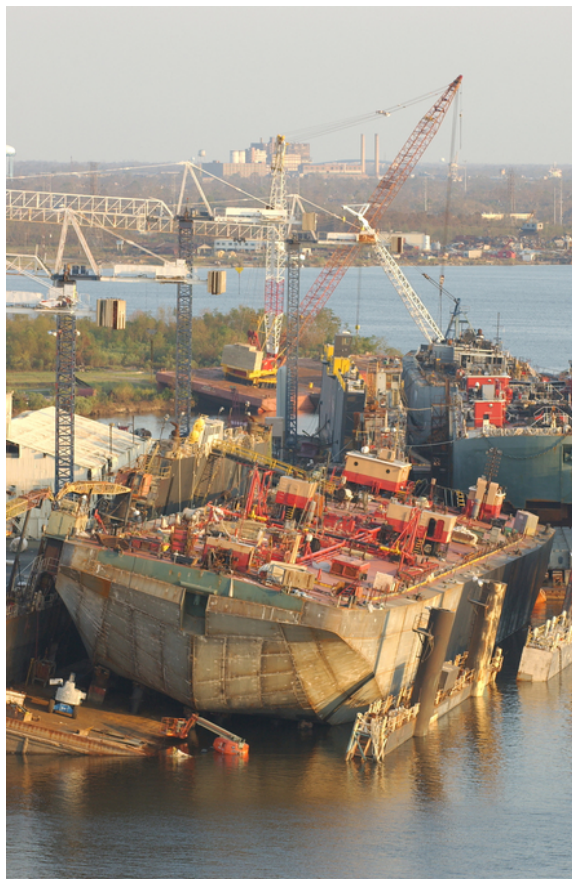
Figure 6: A large ship is forced against the port structure in New Orleans.
