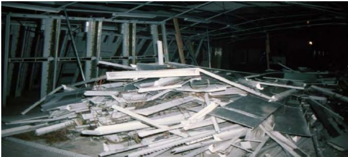
Figure 8-4. Light Fixture and Equipment Failure inside Central Office in Mexico City 1985 Earthquake (OSSPAC 2013)
