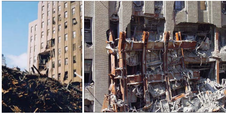
Figure 8-2. Damage to Verizon Building on September 11, 2001 (FEMA 2002)
