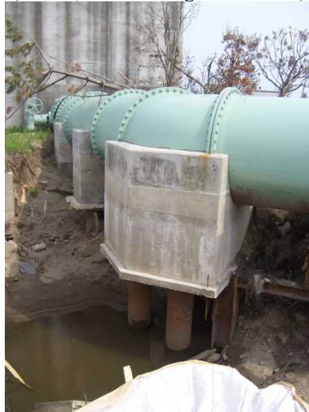
Figure 9.26 Collapse of pipe rack next to digesters due to tsunami scour, Tohoku earthquake, Japan, 2011 (Source: Tang & Edwards, 2014)
