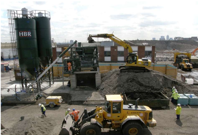
Treatment of soil washing residues, Olympic Park
