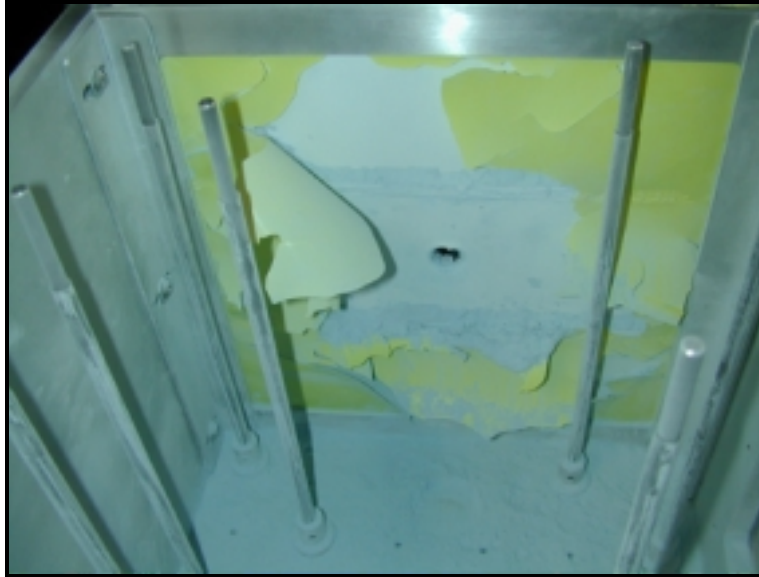
Figure 5-1. Test Example of Significant Panel Fracture and Material Loss
