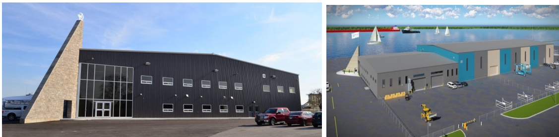
Figure 1: A) Front view of the Hamilton Port Authority boat storage facility used to host the event. It was mostly empty for the summer. B) Back view of the same facility. They also provided dock space in the Lake Ontario to embed our underwater test methods to conduct trials in the opaque water more typically associated with response operations.
