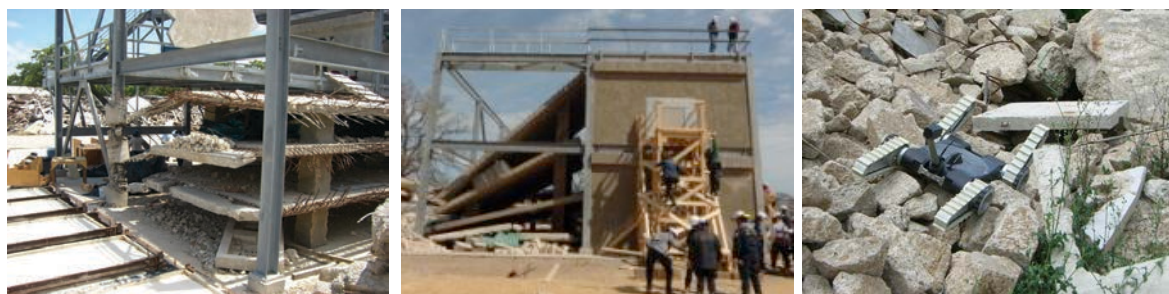
FIGURE 34: Conduct confined space and rubble pile searches.
