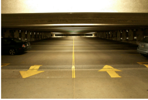
Figure 7: Before LED Lighting Deployment
