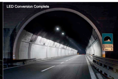
Figure 11: LED Conversion Complete
