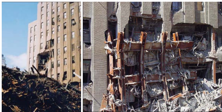
Figure 8-2. Damage to Verizon Building on September 11, 2001 (FEMA 2002)
