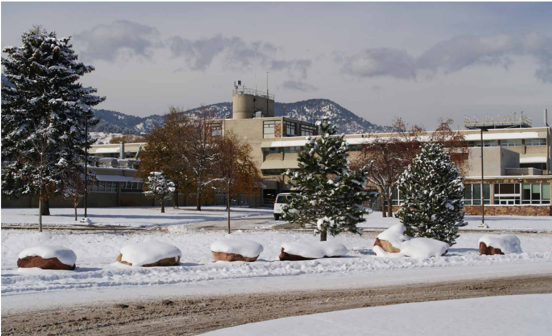
Building 1: Radio Building
