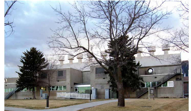
Building 3: Liquifier Building
