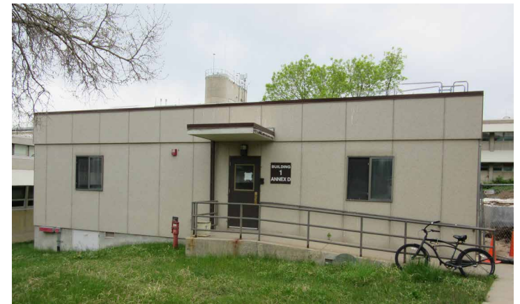
Building 1D: Annex
