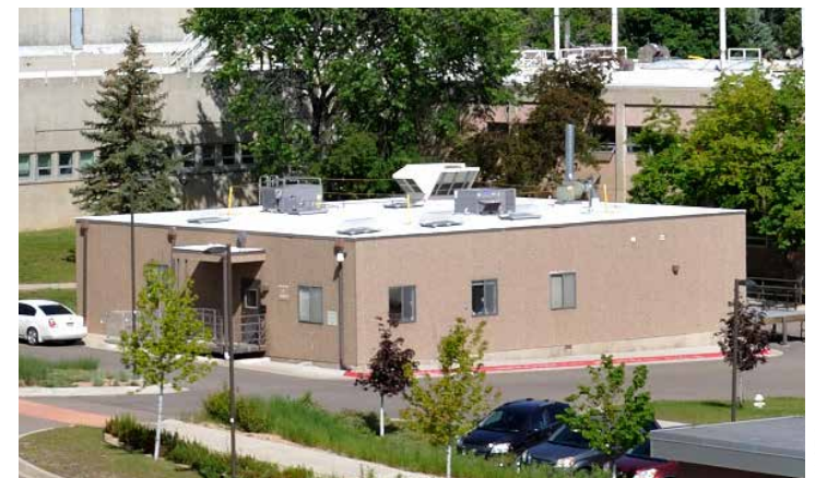
Building 2A: Cryogenic Annex
