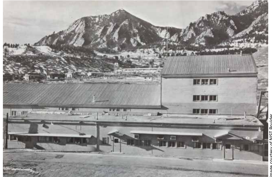
1967 Photograph of Building 4, looking southwest
