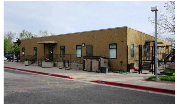
Building 26: Childcare Center
