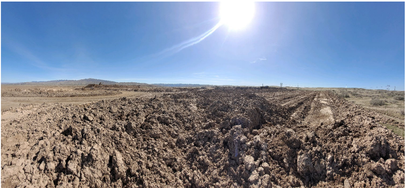
Figure 8. Panorama View of Ongoing Excavations within the APE.
