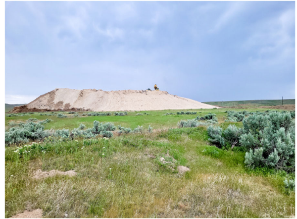
Figure 10. Spoils Pile in the Eastern Portion of the APE, Heavy Equipment on Top is Approximately 20 ft. Tall.
