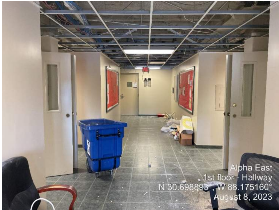
Photograph 5 – Alpha East – 1 st Floor Interior.
