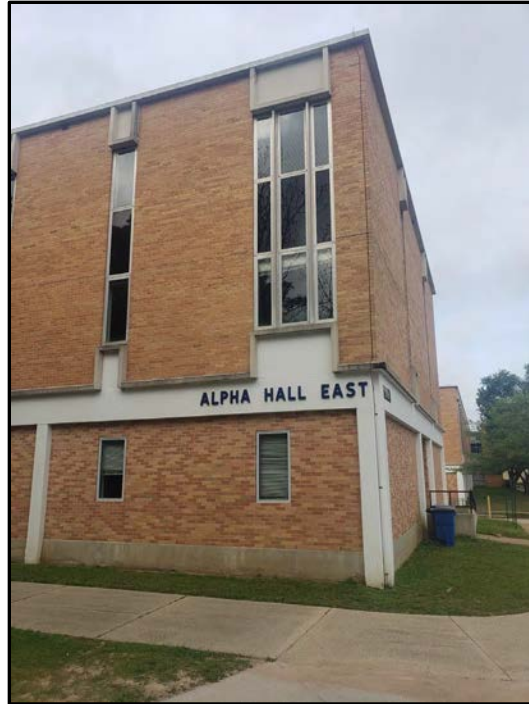
Figure 8. Alpha Hall East, to be demolished.
