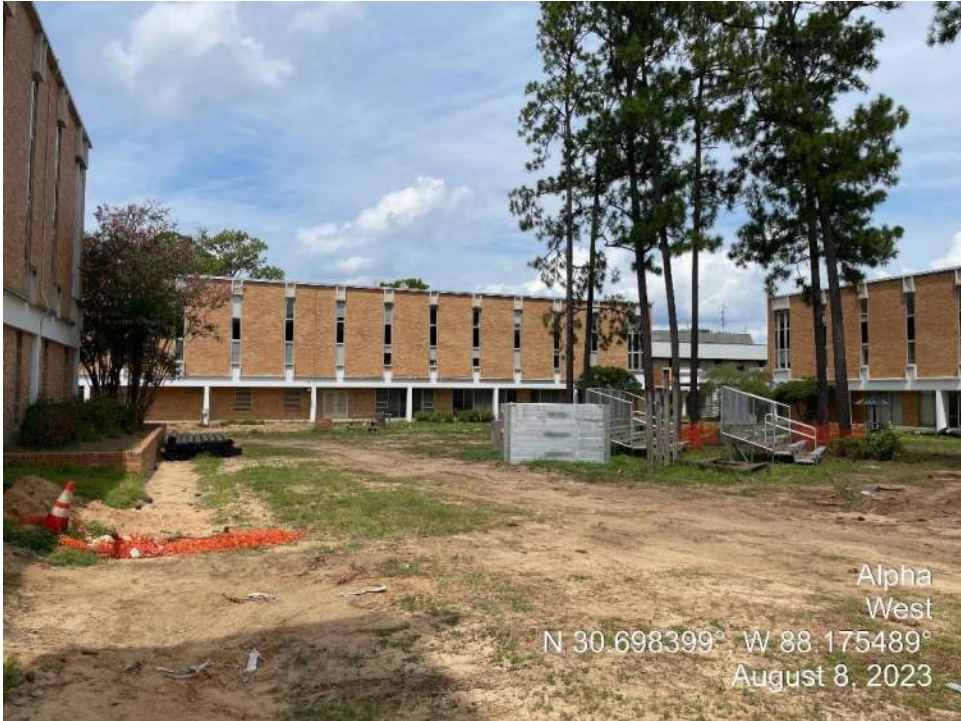
Photograph 23 – Adjacent properties to the west.
