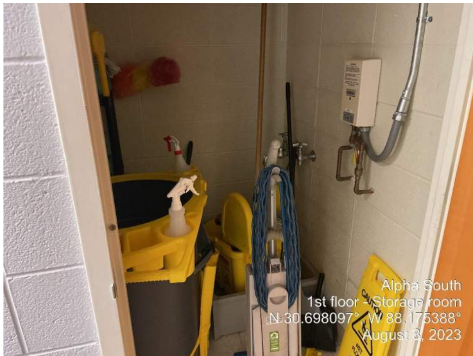
Photograph 16 – Alpha South – Janitorial Storage Room.
