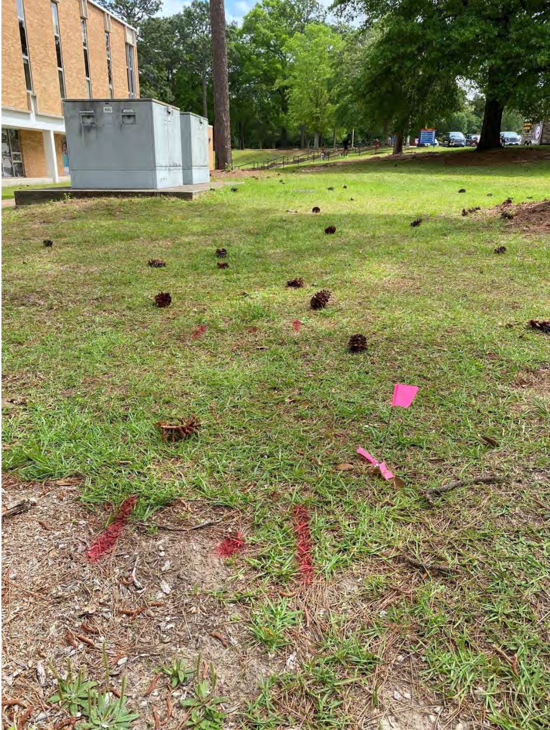
Figure 7. Above ground utilities, marked utilities, and a potential shovel test location along Transect 3 facing east, Alpha Hall South shown in upper left.
