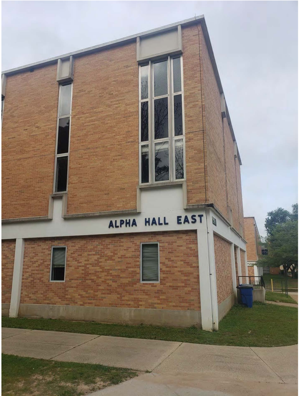
Figure 3. Alpha Hall East northeast corner.
