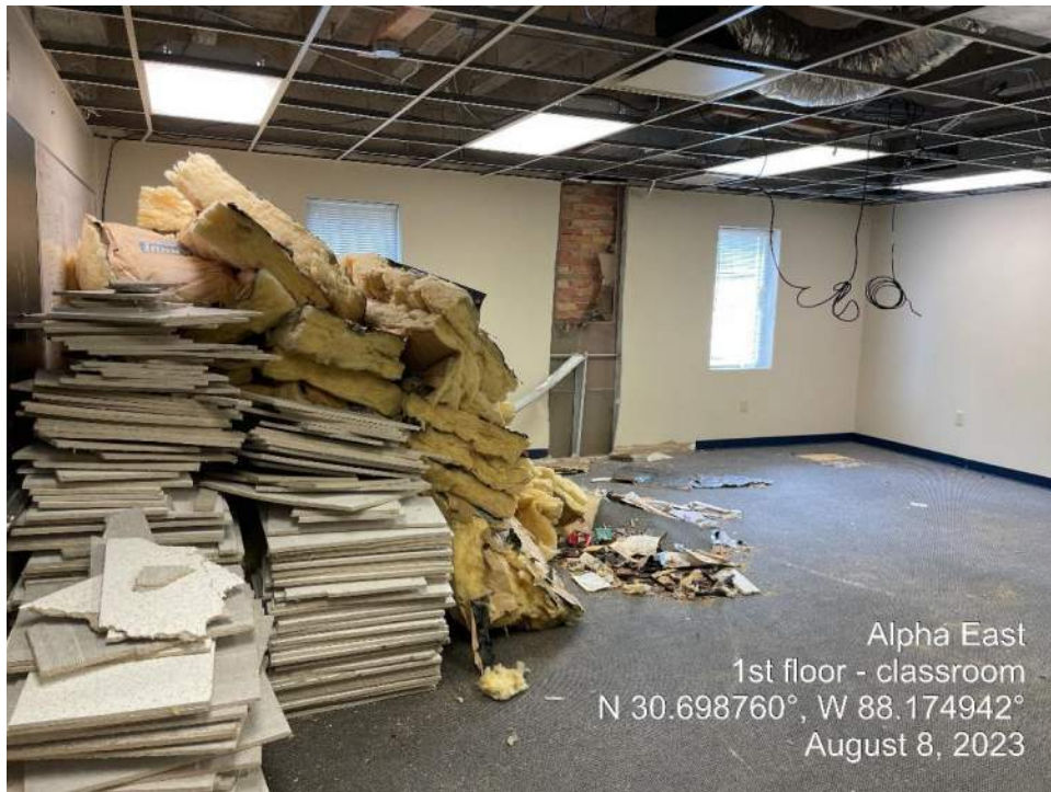
Photograph 6 – Alpha East – 1 st Floor Classroom.
