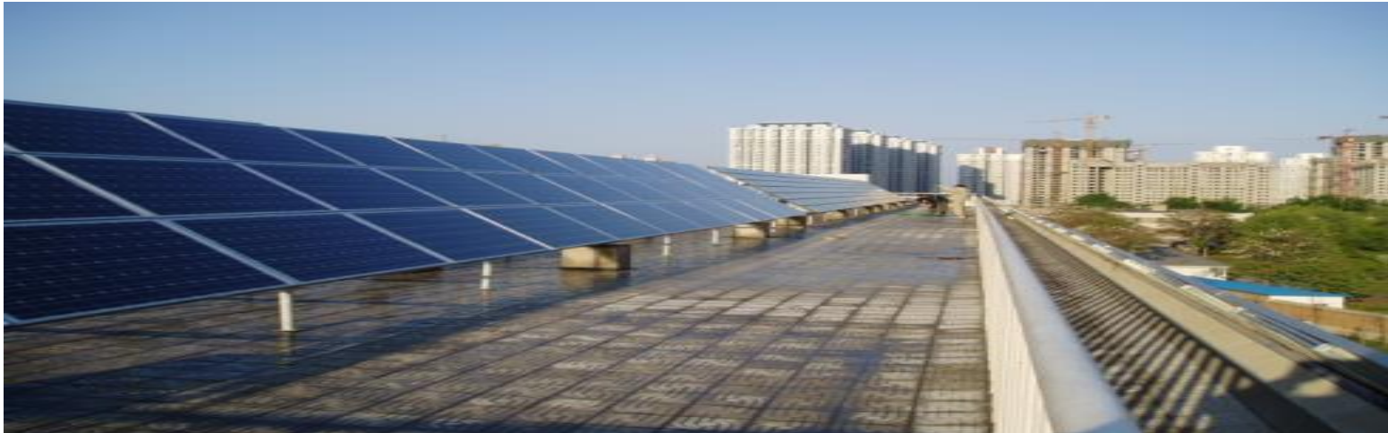
18yrs field module with TPT backsheet shows low power loss rate (0.7%/yr)
