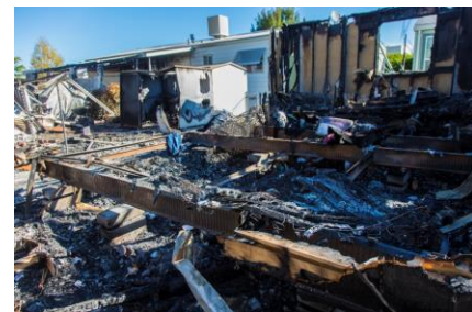
Figure 6-10: Fire damage from broken gas lines (Photographer: Christopher Mardorf, 2014)
