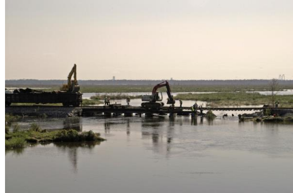
Figure 6-4: A railroad bridge in New Orleans is washed out by flooding (Photo by Marvin Nauman)
