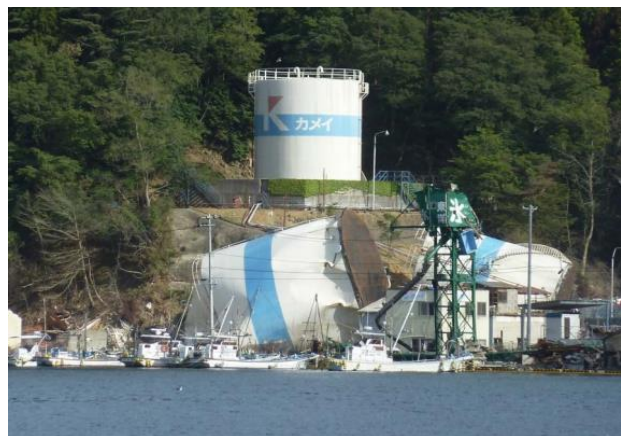
Figure 9-7. Steel Tanks Damaged Due to Tohoku, Japan Tsunami in 2011 (Tang & Edwards 2014)
