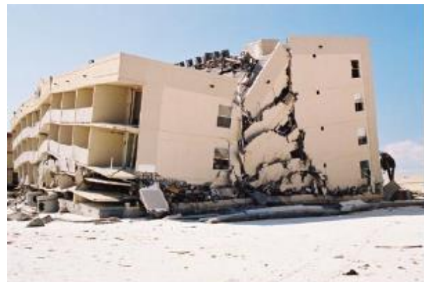
Figure 5-12: Collapse of 5-story building due to undermining (from flooding) of shallow foundation (courtesy of FEMA)
