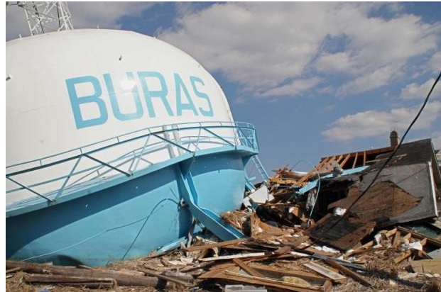
Figure 9-6. Collapsed Water Tank in Buras, LA near Hurricane Katrina Landfall Location (Courtesy of David Goldbloom- Helzner)
