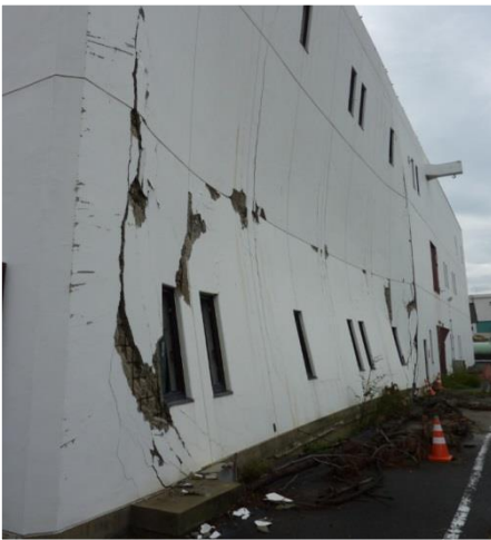
Figure 9-14. Sendai WWTP Effluent Pump Station Damaged by Tsunami in 2011 Tohoku Earthquake (Courtesy of Donald Ballantyne)
