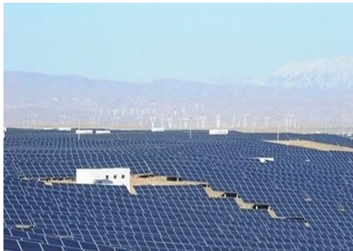
Longyangxia Dam Solar Park, 850MW, China
