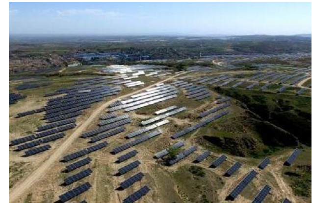
Datong Solar Power Top Runner Base, 1.0 GW, China
