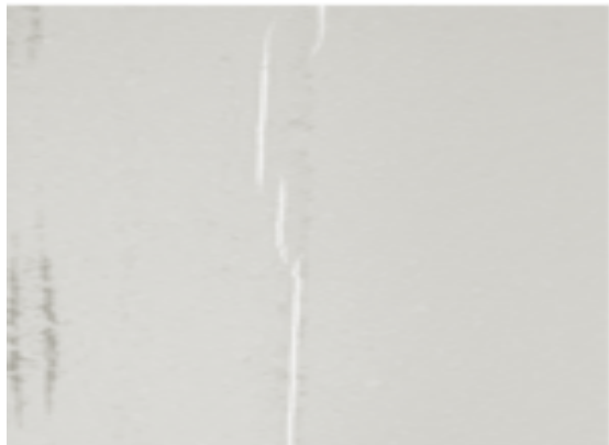
Cracking in 1s PVDF Backsheet
