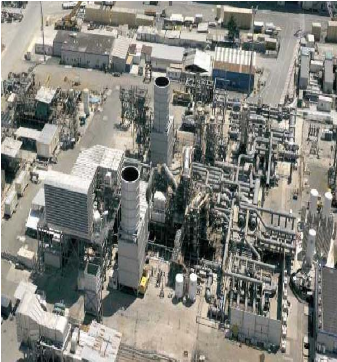
World Largest LNG Train from GE (8 MTPY) tested in Massa, Italy
