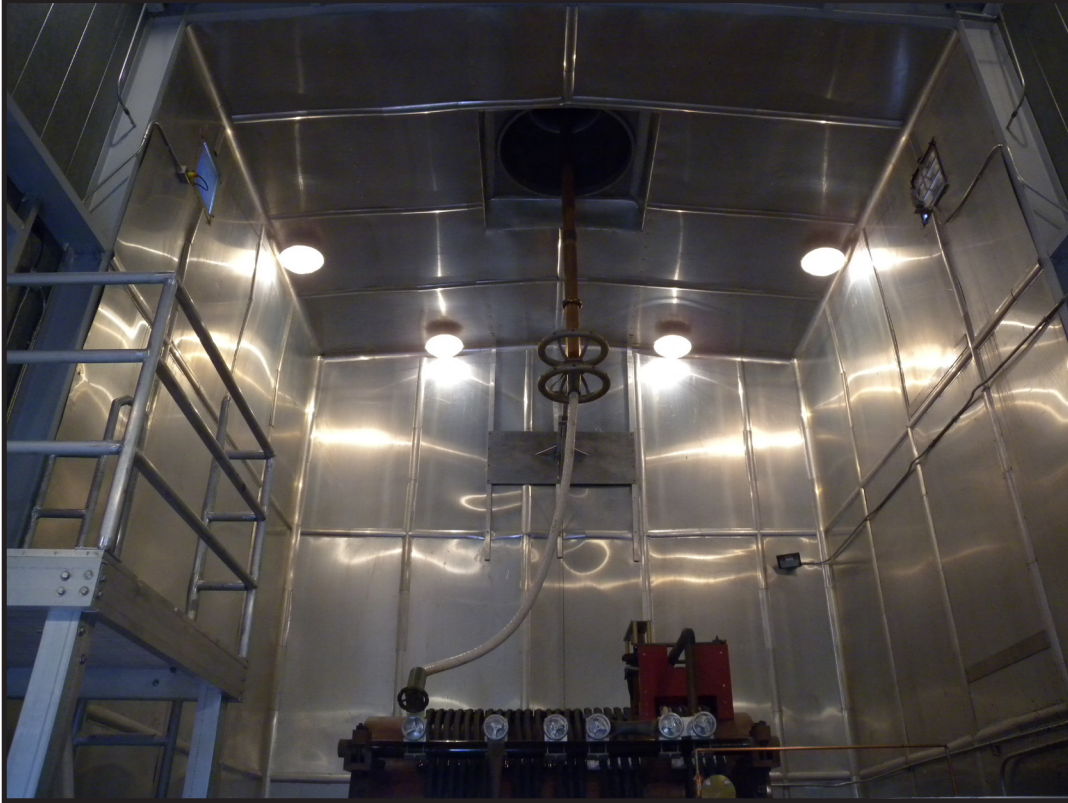
Figure 4.3: Interior of the South Helix House at Fort Collins, Colorado, facing south. August 2019.
