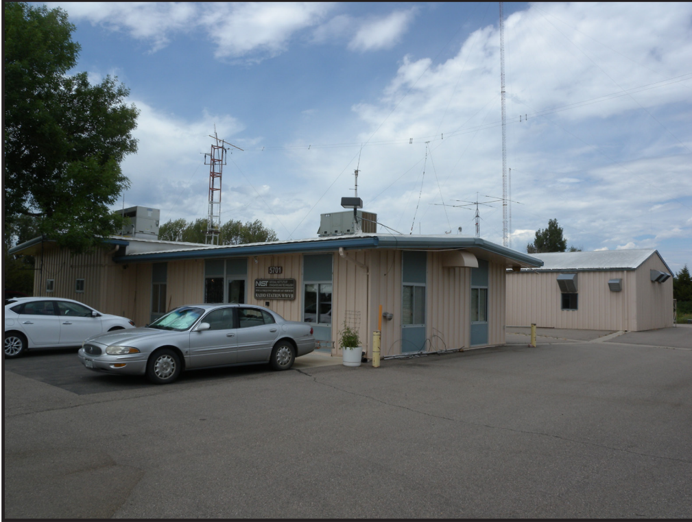
Figure 4.1: Radio Station WWVB at Fort Collins, Colorado, facing northwest. August 2019.
