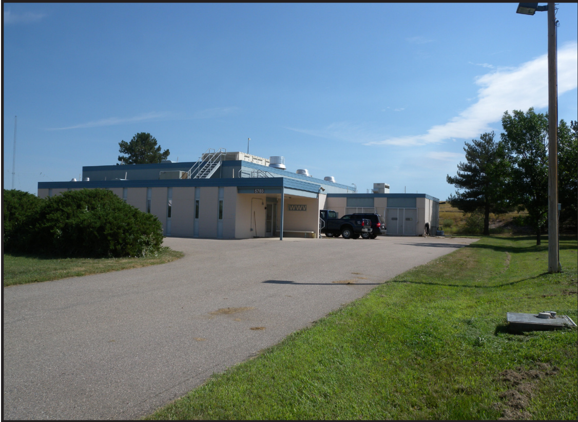
Figure 4.5: Radio Station WWV at Fort Collins, Colorado, facing northeast. August 2019.
