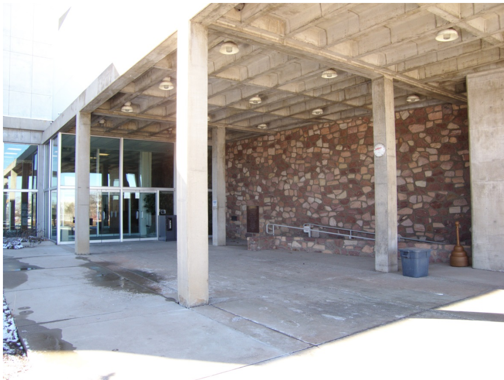
5BL8240:06 Building 1, looking southwest
