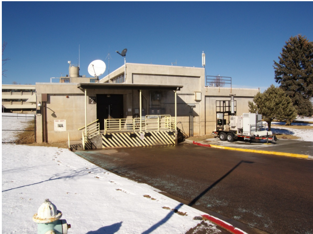
5BL8240:10 Building 1, Wing 2, looking northwest
