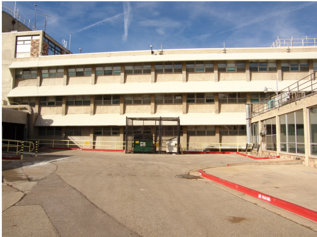
5BL8240:08 Building 1, Spine, looking northwest
