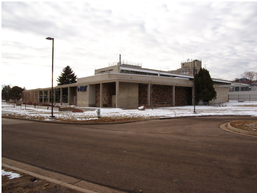
5BL8240:02 Building 1, looking southeast
