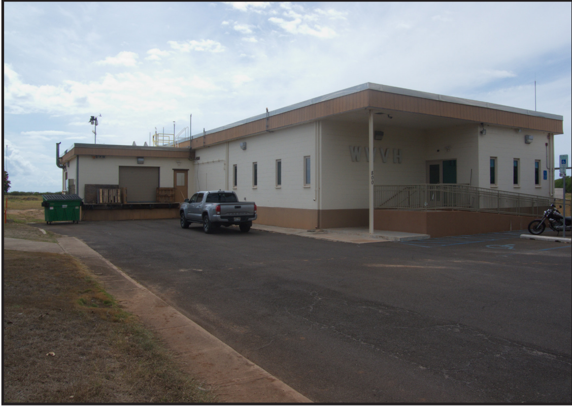
Figure 4.7: Radio Station WWVH at Kekaha, Hawaii, facing west. September 2019.
