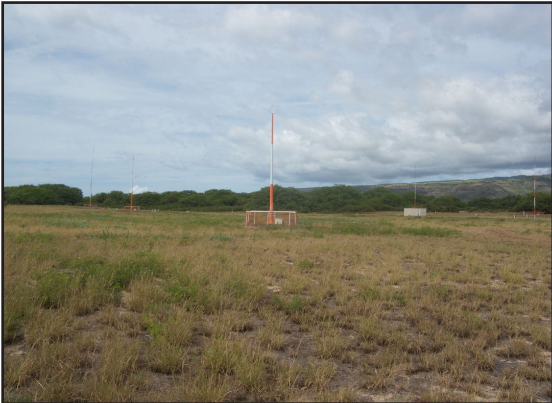
Figure 4.8: WWVH Antenna Systems at Kekaha, Hawaii, facing north. September 2019.
