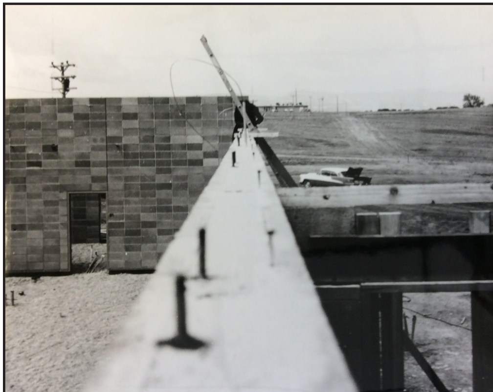
Figure 3.2: Construction of Radio Station WWV at Fort Collins, Colorado, 1966 (courtesy of NIST Fort Collins).
