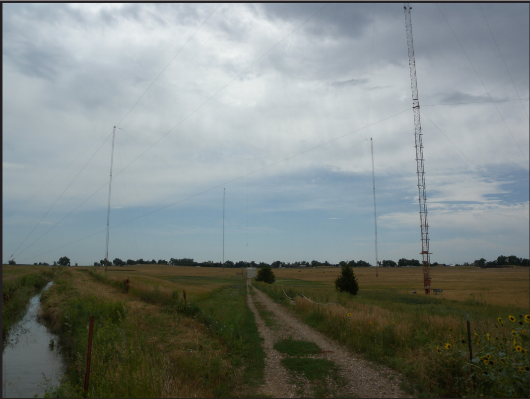
Figure 4.4: South Helix House and Antenna Structures at Fort Collins, Colorado, facing south. August 2019.
