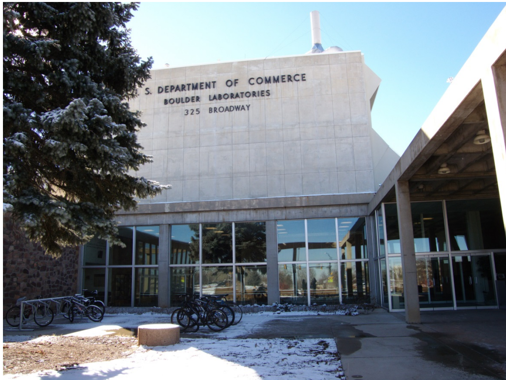
5BL8240:01 Building 1, looking southwest
