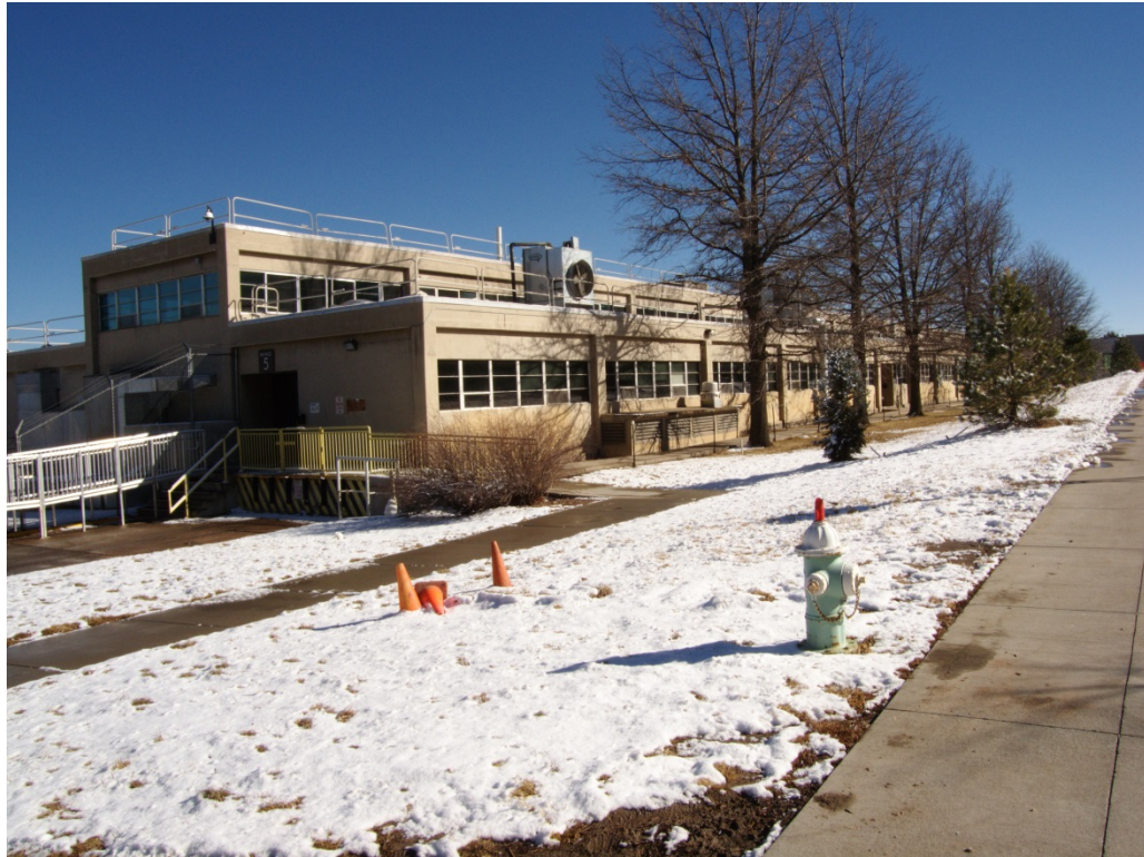
5BL8240:09 Building 1, Wing 5, looking northeast
