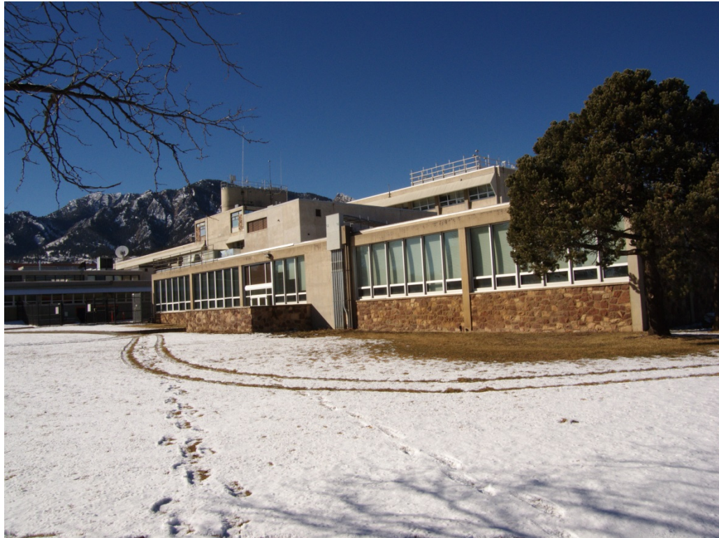
5BL8240:07 Building 1, looking west
