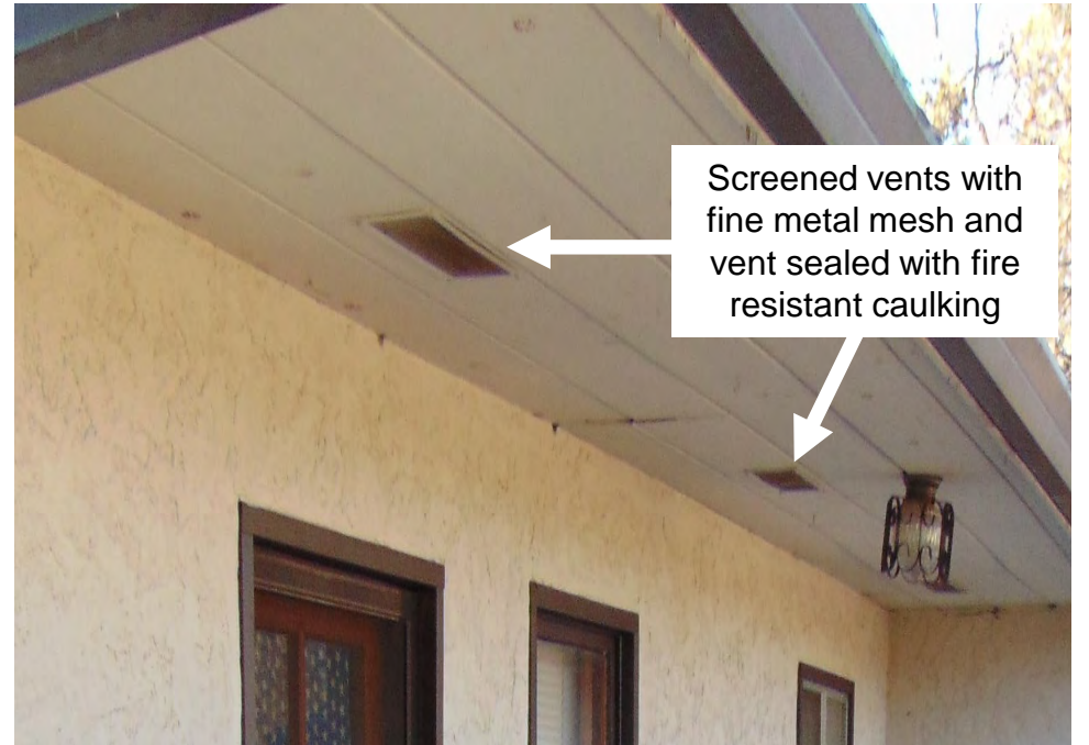
Screened vent with fine metal mesh and vent sealed with fire resistant caulking
