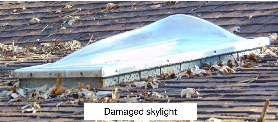
Damaged skylight
