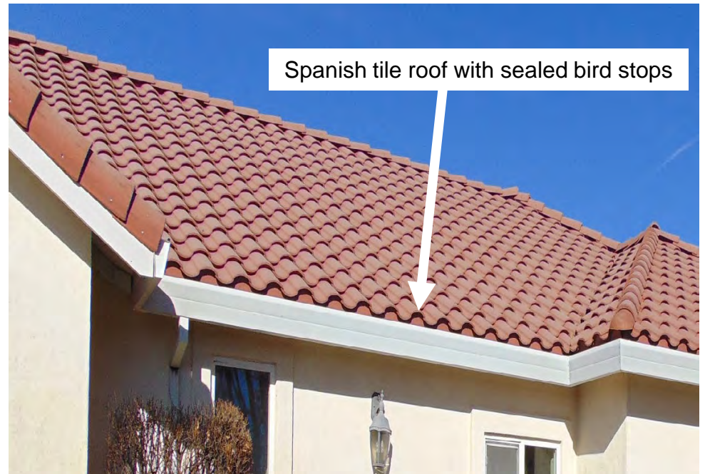
Item 6 Roof Covering (Classes B and C) – Hardened roof materials like metal and Spanish tile prevent ignition.
