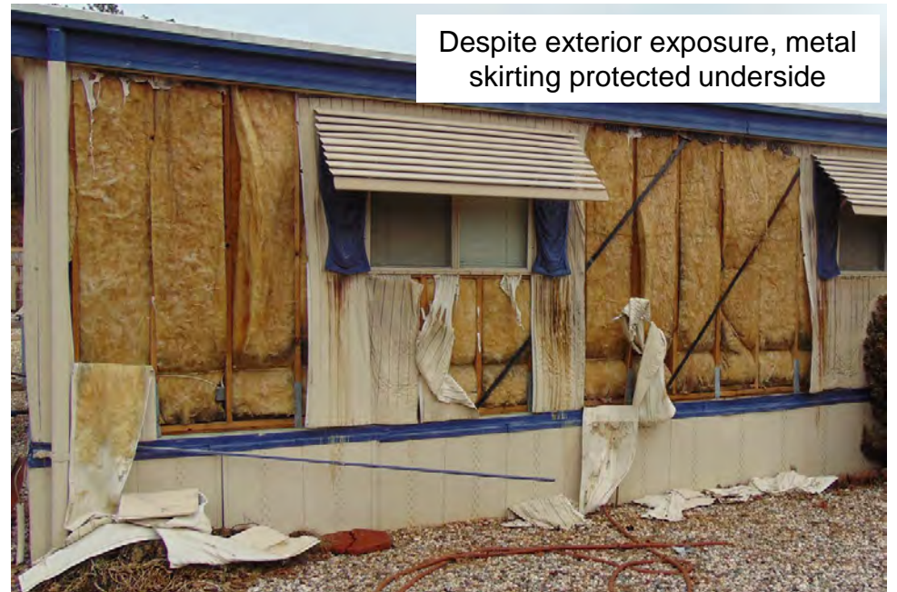
Item 37 Mobile Home Skirting – Noncombustible skirting can prevent mobile home underside from igniting and accumulating flammable (windblown) debris.
