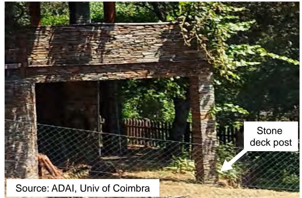
Item 10 Height of Wall Assembly – Hardening exterior walls and deck supports 2 ft above ground will prevent windblown debris and embers from igniting the wall.
