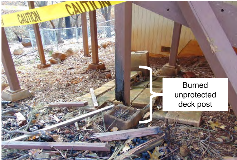
Item 10 Height of Wall Assembly – Hardening exterior walls and deck supports 2 ft above ground will prevent windblown debris and embers from igniting the wall.
