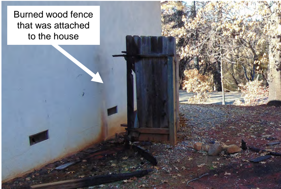
Item 31 Fence Attached to Residence – Keep combustible fence away from house, use noncombustible fence within 8 ft of house.
