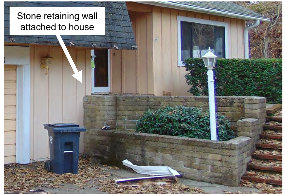
Brick retaining wall attached to house
