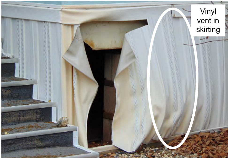
Item 39 Crawl Space Vents – Keep vents clean and covered with a 1/8 th inch fine metal mesh screen to prevent ember intrusion.
