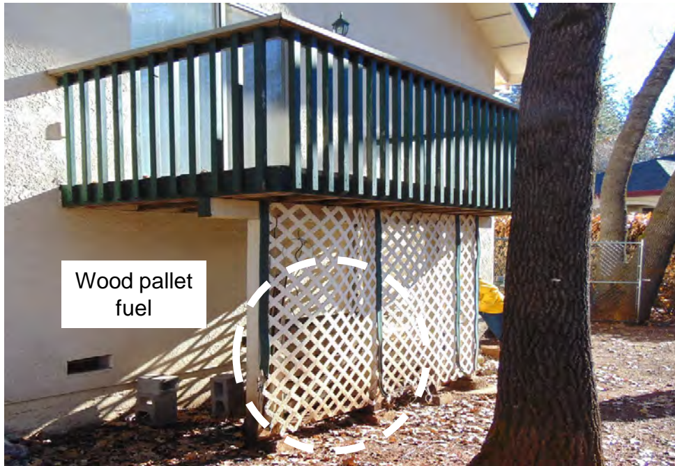
Item 30 Combustible Decks & Nearby Fuels – Remove combustibles around the house and away from the deck.
