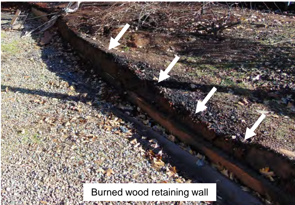
Burned wood retaining wall
