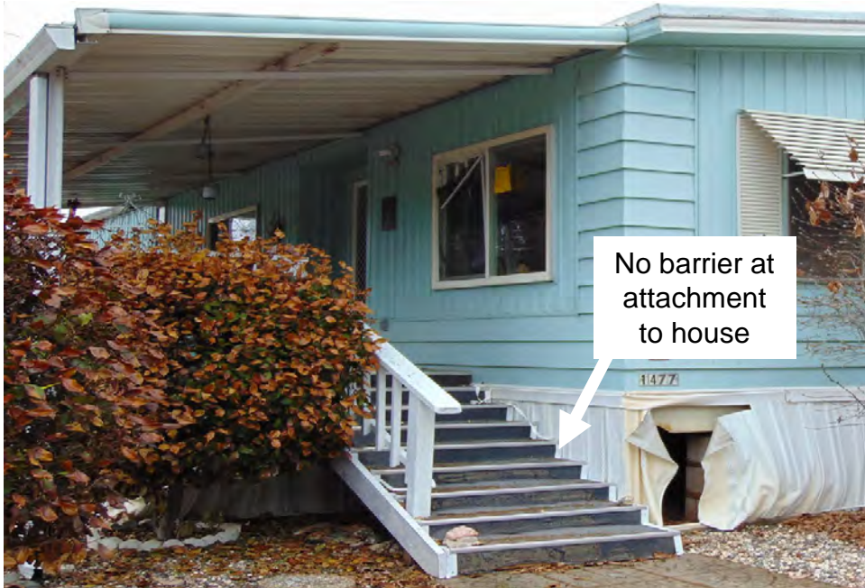
Item 19 Other Attachments to Mobile Home – Noncombustible barrier between mobile home attachments and house exterior.
