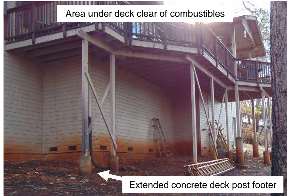
Item 30 Combustible Decks & Nearby Fuels – Remove combustibles around the house and away from the deck.
