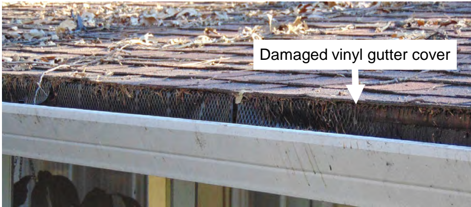
Damaged vinyl gutter cover
