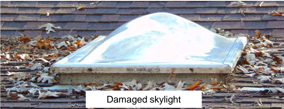
Damaged plastic skylights
