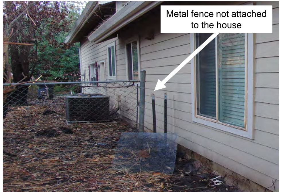
Item 31 Fence Attached to Residence – Keep combustible fence away from house, use noncombustible fence within 8 ft of house.
