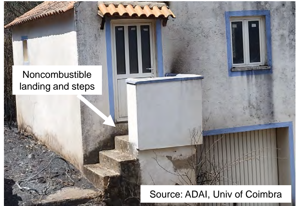
Noncombustible deck with concrete steps and metal rail
