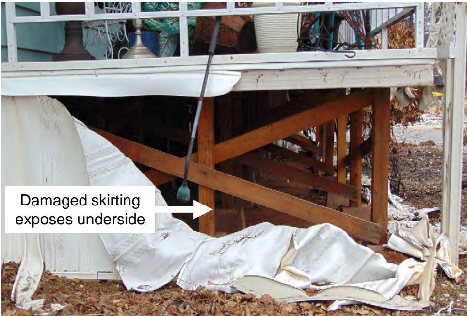
Item 37 Mobile Home Skirting – Noncombustible skirting can prevent mobile home underside from igniting and accumulating flammable (windblown) debris.
