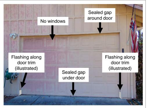
Item 27 Garage Door – Sealed garage doors with metal flashing along lower frame can reduce risk of garage ignition.
