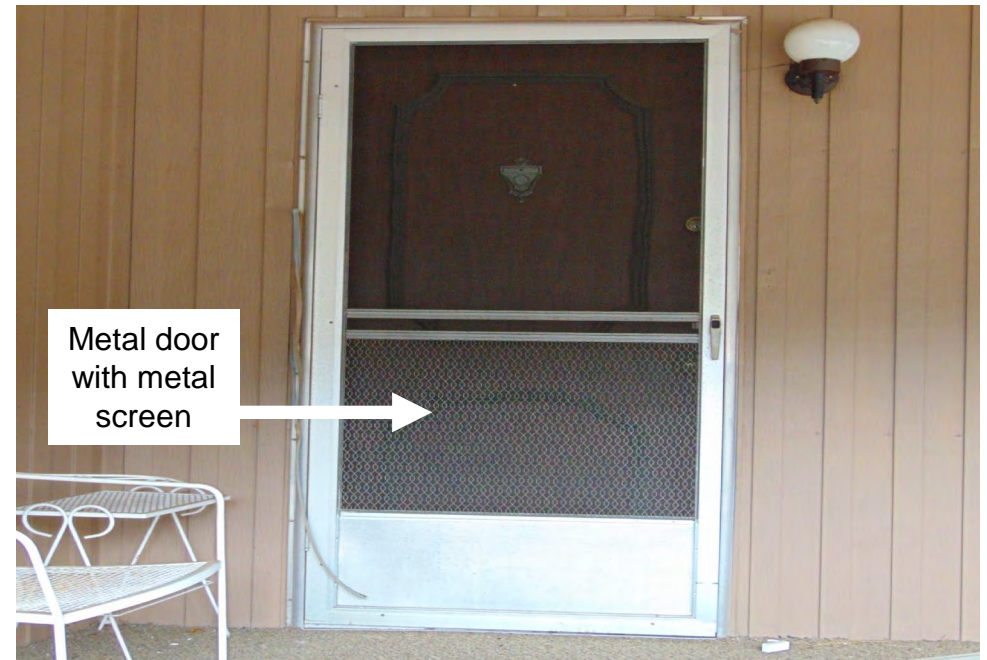
Item 26 Plastic Screen Door – Replace plastic screen doors with metal screens and doors to reduce ignition risk.
