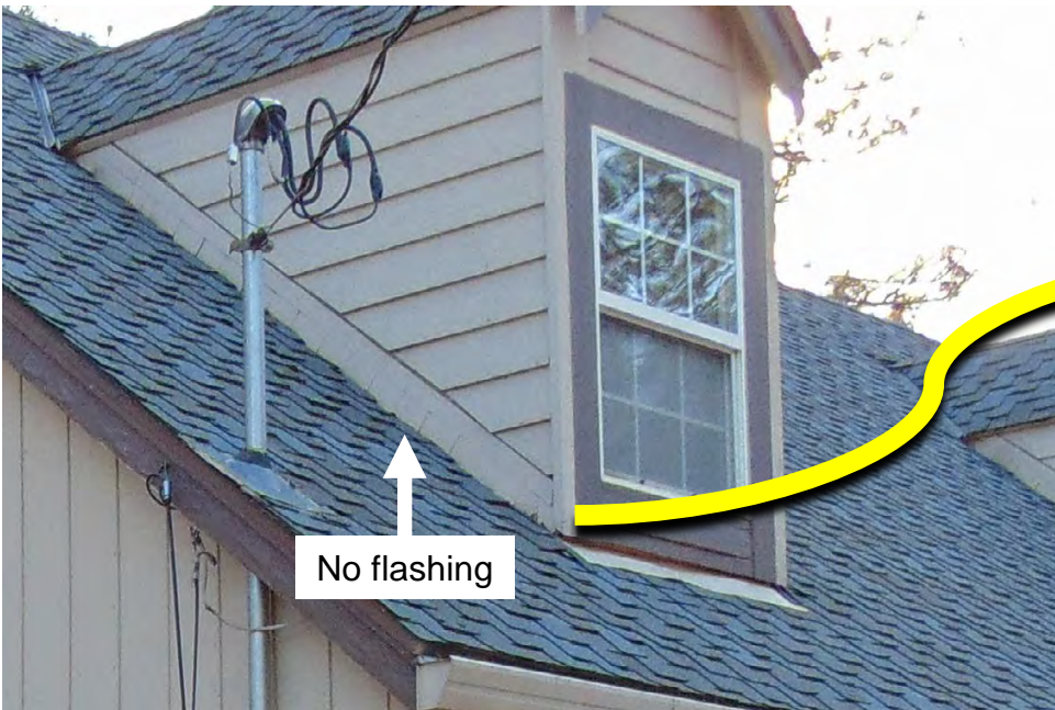
Item 3.2 Roof Assembly Details (Dormers) – Flashing and ignition resistant siding to protect dormer from ignition by combustible debris and embers.
