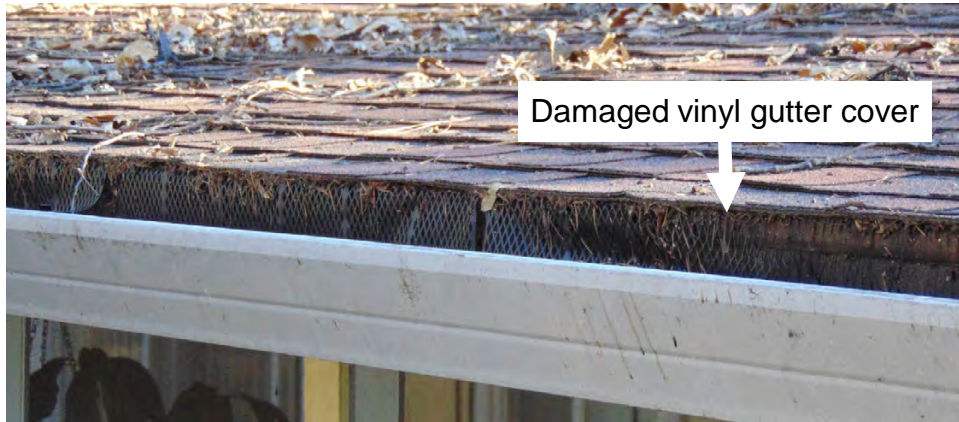
Damaged vinyl gutter cover
